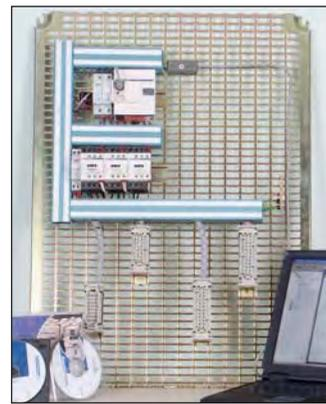
Wired door plate and grid for system operation with a Twido PLC. Supplied with programming and training software.
