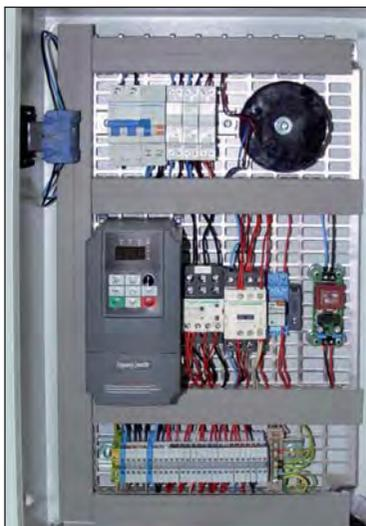
Wired grid including with a speed controller
