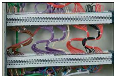
Terminal block built into the cabinet
