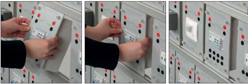
Rapid installation of modules on the frame
